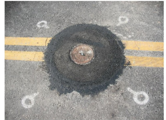
This is a monument well sometimes call a monument box. The 4 small circles are nails used to install the monument well.
