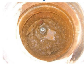
Inside the monument well there is a 3/4 inch iron pipe with a brass tag.
